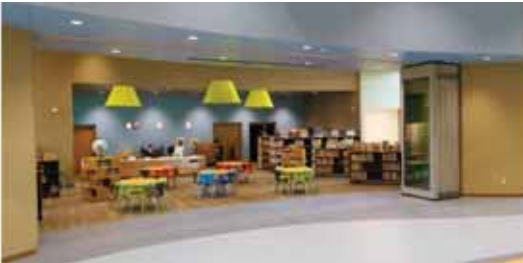
Floor area increased by opening an acoustical glass wall partition with manual and/or automatic operation
