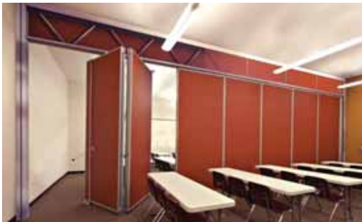
Unispan installed with header panels below ceiling height.
